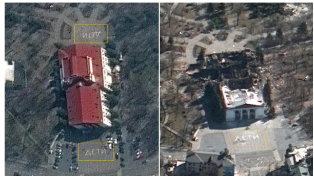
Figure 1 Mariupol Theatre: Before and After
